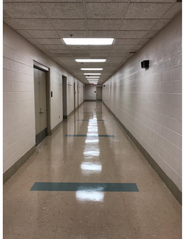
Sample Guard Equipment Storage Hallway
